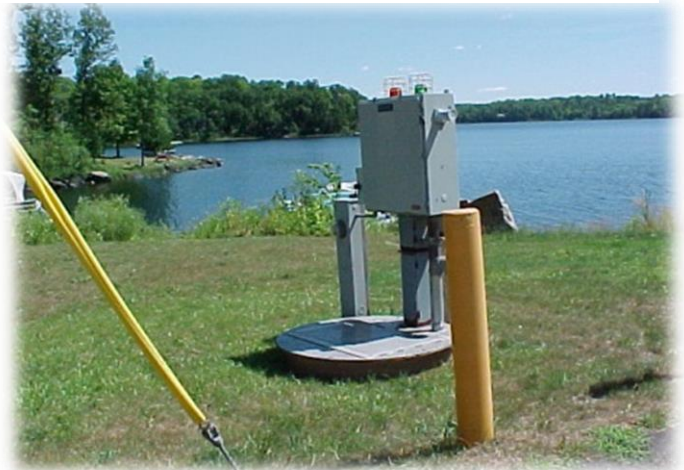
FIGURE 26 LIFT STATIONS ON THE SHORE OF LAKE MICHIGAMME
