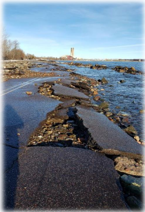
FIGURE 8 SHORLINE EROSION ON LAKESHORE BOULEVARD IN MARQUETTE
